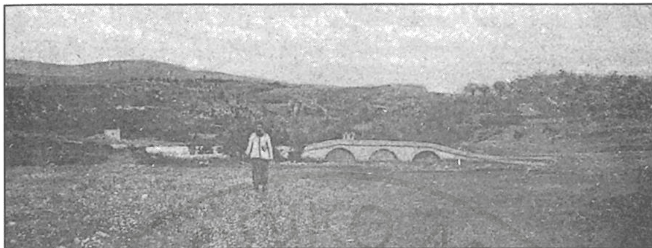
Vrysses - The bridge
