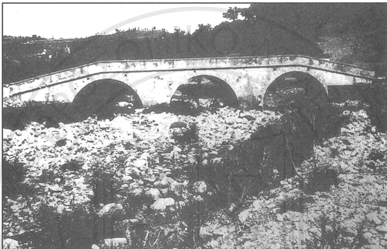
The bridge of Vrysses
